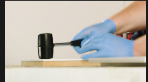
Tap lightly with a mallet to secure the bond.
